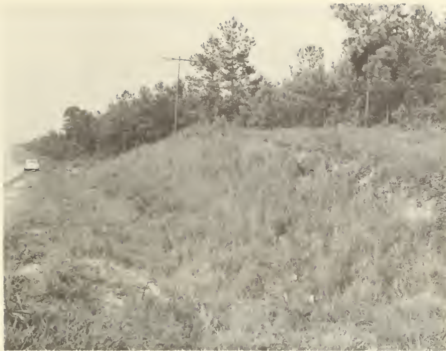
Figure 20.--Broomsedge straw, cut from adjacent field areas in October when full of mature seed, was lightly mulched on this roadbank. In May, after seeding and when stands were up, fertilization preserved the stand.
